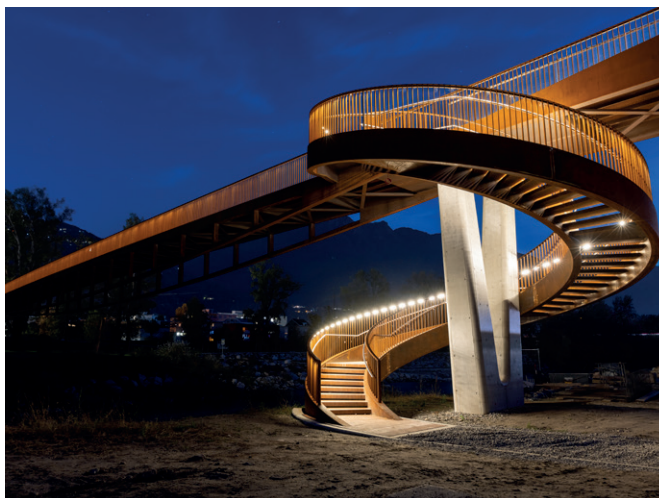
LaneLED WALL, Passerella Torretta Bellinzona
